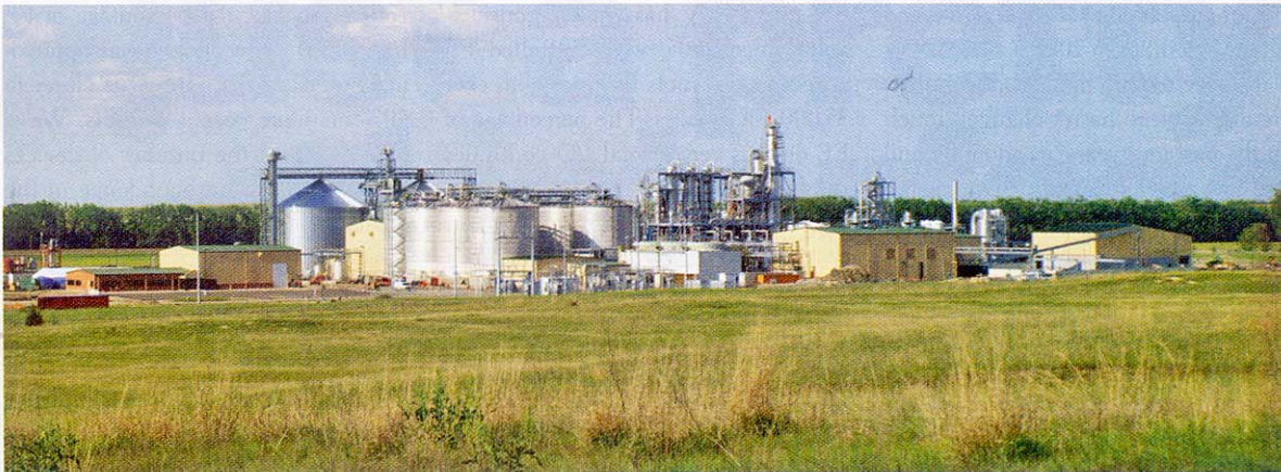
Figure 1: Abengoa Bioenergy's new plant in Ravenna, Neb., uses a dry-mill process to produce ethanol from corn starch with help from Foundation fieldbus, Profibus and AS-i protocols.
